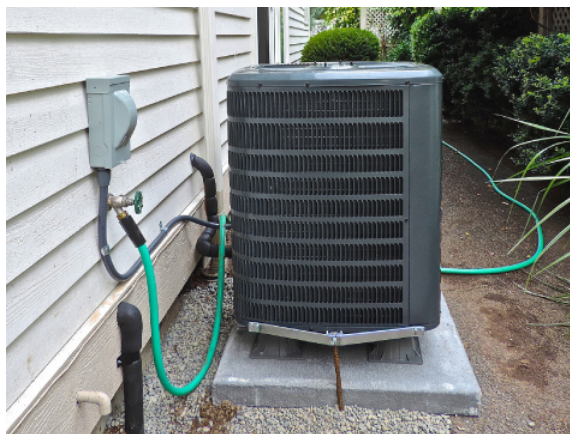
Figure 14.16.4. A photograph of a heat pump (large box) located outside a house. This heat pump is located in a warm climate area, like the southern United States, since it would be far too inefficient located in the northern half of the United States. (credit: modification of work by Peter Stevens).
