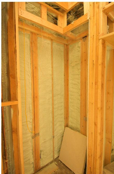
Figure 2: Insulation is used to limit the conduction of heat from the inside to the outside (in winter) and from the outside to the inside (in summer). (credit: Giles Douglas)
