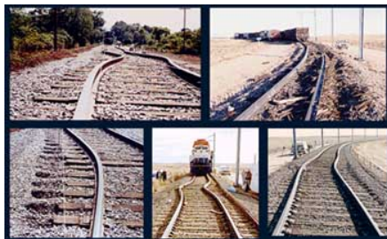
Fig 1: Thermal expansion of long continuous sections of rail tracks is the driving force for rail buckling. This phenomenon resulted in 190 train derailments during 1998–2002 in the US alone.
