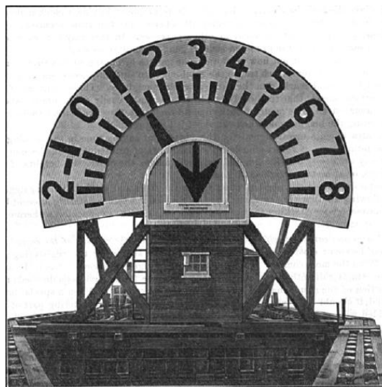
FIG. 5.—Tidal indicator, Delaware River, Delaware.
