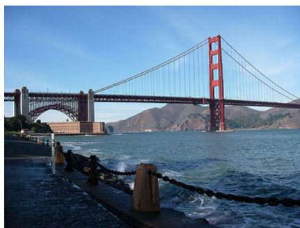
Figure 4.6.9: Unless an infinite tension is exerted, any flexible connector—such as the chain at the bottom of the picture—will sag under its own weight, giving a characteristic curve when the weight is evenly distributed along the length. Suspension bridges—such as the Golden Gate Bridge shown in this image—are essentially very heavy flexible connectors. The weight of the bridge is evenly distributed along the length of flexible connectors, usually cables, which take on the characteristic shape. (credit: Leaflet, Wikimedia Commons)
