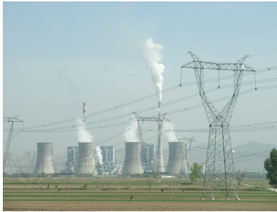
Figure 6.8.3: Tremendous amounts of electric power are generated by coal-fired power plants such as this one in China, but an even larger amount of power goes into heat transfer to the surroundings. The large cooling towers here are needed to transfer heat as rapidly as it is produced. The transfer of heat is not unique to coal plants but is an unavoidable consequence of generating electric power from any fuel—nuclear, coal, oil, natural gas, or the like. (credit: Kleinolive, Wikimedia Commons)
