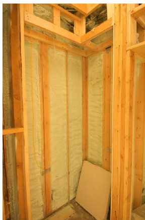
Figure 8.6.1: Insulation is used to limit the conduction of heat from the inside to the outside (in winters) and from the outside to the inside (in summers). (credit: Giles Douglas)
