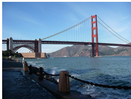
Figure 4.6.9: Unless an infinite tension is exerted, any flexible connector—such as the chain at the bottom of the picture—will sag under its own weight, giving a characteristic curve when the weight is evenly distributed along the length. Suspension bridges—such as the Golden Gate Bridge shown in this image—are essentially very heavy flexible connectors. The weight of the bridge is evenly distributed along the length of flexible connectors, usually cables, which take on the characteristic shape. (credit: Leaflet, Wikimedia Commons)
