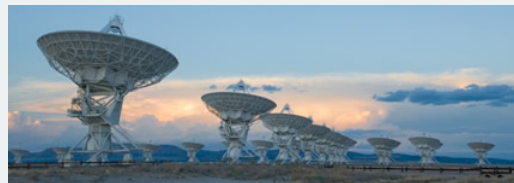
Figure B.9 Radio telescopes in the Very Large Array (VLA). These antennas are located in New Mexico. The signals from the antennas are combined, or synthesized, to effectively create a single telescope with much higher resolution than any single dish. Click on the image to learn more. Credit: courtesy of NRAO/AUI and NRA.
