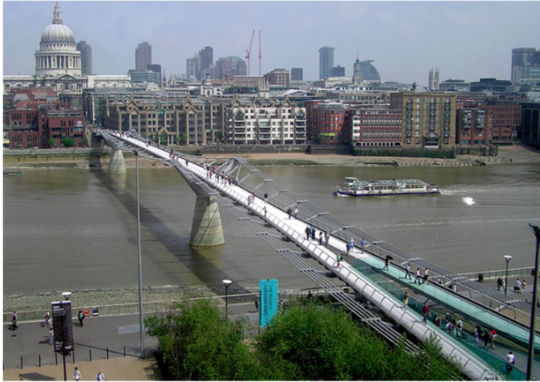
Figure 15.7.6: Initially when people crossed the London Millennium Footbridge, they experienced a swaying motion. People continuing to cross reinforced the oscillation's amplitude, thereby increasing the problematic swaying. (credit: Adrian Pingstone/Wikimedia Commons)
