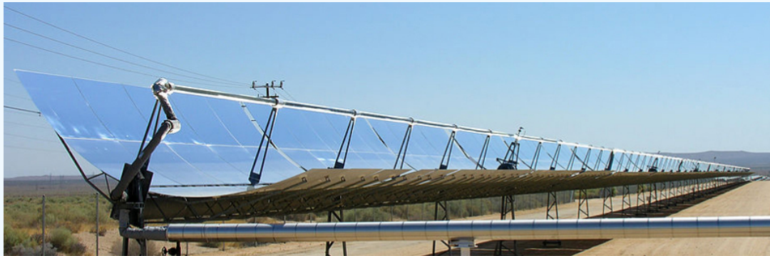
Figure 11.3.7: Parabolic trough collectors are used to generate electricity in southern California. (credit: “kjkolb”/Wikimedia Commons)
