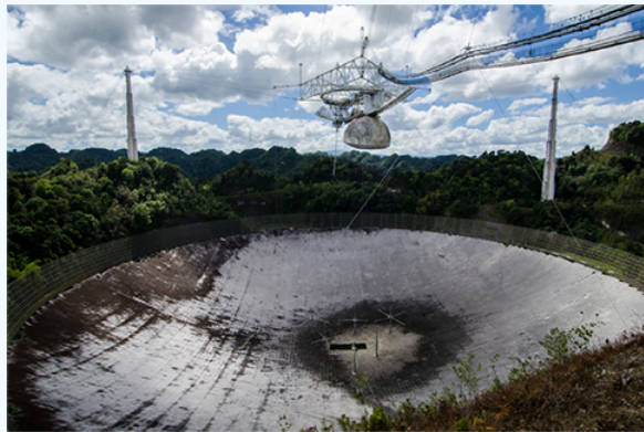
Figure 14.6.4: A 305-m-diameter paraboloid at Arecibo in Puerto Rico is lined with reflective material, making it into a radio telescope. It is the largest curved focusing dish in the world. Although D for Arecibo is much larger than for the Hubble Telescope, it detects radiation of a much longer wavelength and its diffraction limit is significantly poorer than Hubble's. The Arecibo telescope is still very useful, because important information is carried by radio waves that is not carried by visible light. (credit: Jeff Hitchcock)
