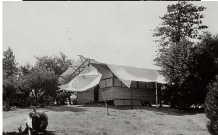
Figure 2.7.3 - Dayton Miller thought that the result of the Michelson-Morley experiment could be explained because the ether had been pulled along by the dirt, and the walls of the laboratory. This motivated him to carry out a series of experiments at the top of Mount Wilson, in a building with thin walls.
