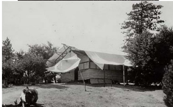
Figure 2.7.3 - Dayton Miller thought that the result of the Michelson-Morley experiment could be explained because the ether had been pulled along by the dirt, and the walls of the laboratory. This motivated him to carry out a series of experiments at the top of Mount Wilson, in a building with thin walls.
