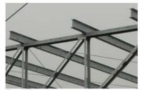
Figure 12.4.4: Steel I-beams are used in construction to reduce bending strains. (credit: modification of work by "US Army Corps of Engineers Europe District"/Flickr)
