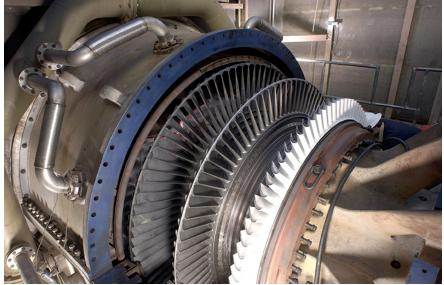
Figure 13.7.5: Steam turbine/generator. The steam produced by burning coal impacts the turbine blades, turning the shaft, which is connected to the generator.
