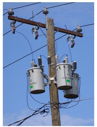
Figure 15.7.2: Transformers are used to step down the high voltages in transmission lines to the 110 to 220 V used in homes. (credit: modification of work by "Fortyseven"/Flickr)
