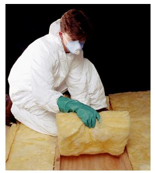
Figure 1.7.5: The fiberglass batt is used for insulation of walls and ceilings to prevent heat transfer between the inside of the building and the outside environment. (credit: Tracey Nicholls)
