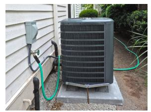
Figure 4.6.4. A photograph of a heat pump (large box) located outside a house. This heat pump is located in a warm climate area, like the southern United States, since it would be far too inefficient located in the northern half of the United States. (credit: modification of work by Peter Stevens).
