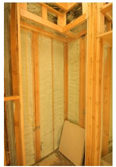
Figure 1.7.2: Insulation is used to limit the conduction of heat from the inside to the outside (in winter) and from the outside to the inside (in summer). (credit: Giles Douglas)
