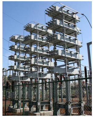
Figure 15.4.4: Power capacitors are used to balance the impedance of the effective inductance in transmission lines.
