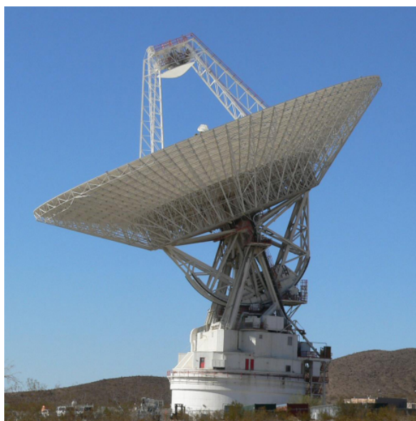
Figure 10.9.2 Radar Telescope. This dish-shaped antenna, part of the NASA Deep Space Network in California’s Mojave Desert, is 70 meters wide. Nicknamed the “Mars antenna,” this radar telescope can send and receive radar waves, and thus measure the distances to planets, satellites, and asteroids.
