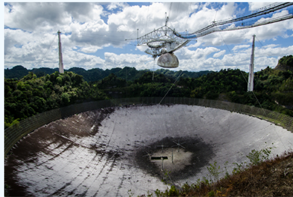
Figure 4.6.4: A 305-m-diameter paraboloid at Arecibo in Puerto Rico is lined with reflective material, making it into a radio telescope. It is the largest curved focusing dish in the world. Although D for Arecibo is much larger than for the Hubble Telescope, it detects radiation of a much longer wavelength and its diffraction limit is significantly poorer than Hubble's. The Arecibo telescope is still very useful, because important information is carried by radio waves that is not carried by visible light. (credit: Jeff Hitchcock)
