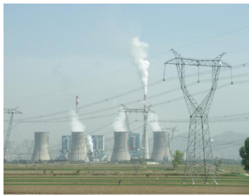
Figure 3.7.3: Tremendous amounts of electric power are generated by coal-fired power plants such as this one in China, but an even larger amount of power goes into heat transfer to the surroundings. The large cooling towers here are needed to transfer heat as rapidly as it is produced. The transfer of heat is not unique to coal plants but is an unavoidable consequence of generating electric power from any fuel—nuclear, coal, oil, natural gas, or the like. (credit: Kleinolive, Wikimedia Commons)
