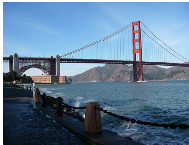
Figure 2.6.4: Unless an infinite tension is exerted, any flexible connector—such as the chain at the bottom of the picture—will sag under its own weight, giving a characteristic curve when the weight is evenly distributed along the length, known as a catenary curve. Suspension bridges—such as the Golden Gate Bridge shown in this image—are essentially very heavy flexible connectors. The weight of the bridge is evenly distributed along the length of flexible connectors, usually cables, which take on the characteristic shape. (credit: Leaflet, Wikimedia Commons)
