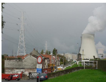
Figure 14.10.1: The people living near this nuclear power plant have no measurable exposure to radiation that is traceable to the plant. About 16% of the world's electrical power is generated by controlled nuclear fission in such plants. The cooling towers are the most prominent features but are not unique to nuclear power. The reactor is in the small domed building to the left of the towers. (credit: Kalmthouts)
