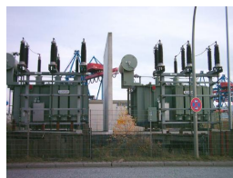
Figure 10.12.4: Power is distributed over large distances at high voltage to reduce power loss in the transmission lines. The voltages generated at the power plant are stepped up by passive devices called transformers to 330,000 volts (or more in some places worldwide). At the point of use, the transformers reduce the voltage transmitted for safe residential and commercial use. (Credit: GeorgHH, Wikimedia Commons)
