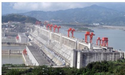
Figure 7.3.2: Three Gorges Dam in central China. When completed in 2008, this became the world's largest hydroelectric plant, generating power equivalent to that generated by 22 average-sized nuclear power plants. The concrete dam is 181 m high and 2.3 km across. The reservoir made by this dam is 660 km long. Over 1 million people were displaced by the creation of the reservoir. (credit: Le Grand Portage)
