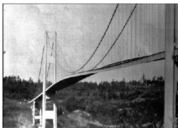
Figure 5.4.4: In 1940, the Tacoma Narrows Bridge in Washington state collapsed. Heavy cross winds drove the bridge into oscillations at its resonant frequency. Damping decreased when support cables broke loose and started to slip over the towers, allowing increasingly greater amplitudes until the structure failed (credit: PRI's Studio 360 , via Flickr)
