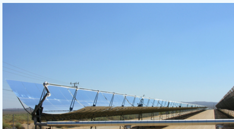
Figure 11.7.5: Parabolic trough collectors are used to generate electricity in southern California. (credit: kjkolb, Wikimedia Commons)
