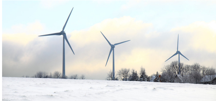
Figure 10.1.1: These wind turbines in the Thames Estuary in the UK are an example of induction at work. Wind pushes the blades of the turbine, spinning a shaft attached to magnets. The magnets spin around a conductive coil, inducing an electric current in the coil, and eventually feeding the electrical grid. (credit: modification of work by Petr Kratochvil)
