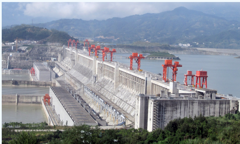
Figure 6.3.2: Three Gorges Dam in central China. When completed in 2008, this became the world's largest hydroelectric plant, generating power equivalent to that generated by 22 average-sized nuclear power plants. The concrete dam is 181 m high and 2.3 km across. The reservoir made by this dam is 660 km long. Over 1 million people were displaced by the creation of the reservoir. (credit: Le Grand Portage)
