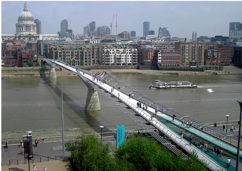
Figure 11.5.6: Initially when people crossed the London Millennium Footbridge, they experienced a swaying motion. People continuing to cross reinforced the oscillation's amplitude, thereby increasing the problematic swaying. (credit: Adrian Pingstone/Wikimedia Commons)
