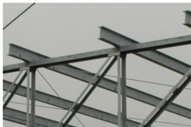
Figure 5.7.4: Steel I-beams are used in construction to reduce bending strains. (credit: modification of work by "US Army Corps of Engineers Europe District"/Flickr)
