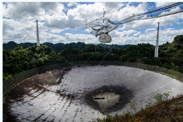
Figure 11.9.4: A 305-m-diameter paraboloid at Arecibo in Puerto Rico is lined with reflective material, making it into a radio telescope. It is the largest curved focusing dish in the world. Although D for Arecibo is much larger than for the Hubble Telescope, it detects radiation of a much longer wavelength and its diffraction limit is significantly poorer than Hubble's. The Arecibo telescope is still very useful, because important information is carried by radio waves that is not carried by visible light. (credit: Jeff Hitchcock)
