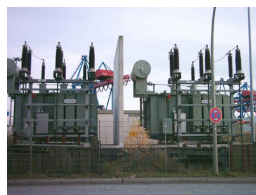
Figure 8.8.4: Power is distributed over large distances at high voltage to reduce power loss in the transmission lines. The voltages generated at the power plant are stepped up by passive devices called transformers to 330,000 volts (or more in some places worldwide). At the point of use, the transformers reduce the voltage transmitted for safe residential and commercial use. (Credit: GeorgHH, Wikimedia Commons)
