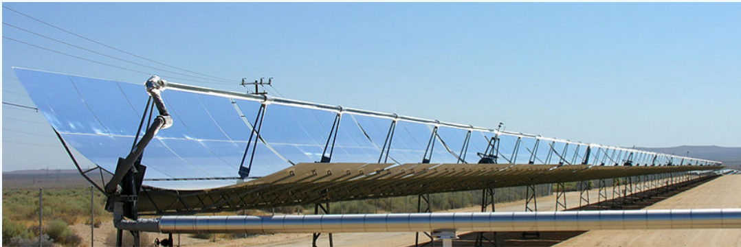
Figure 10.10.7: Parabolic trough collectors are used to generate electricity in southern California. (credit: “kjkolb”/Wikimedia Commons)
