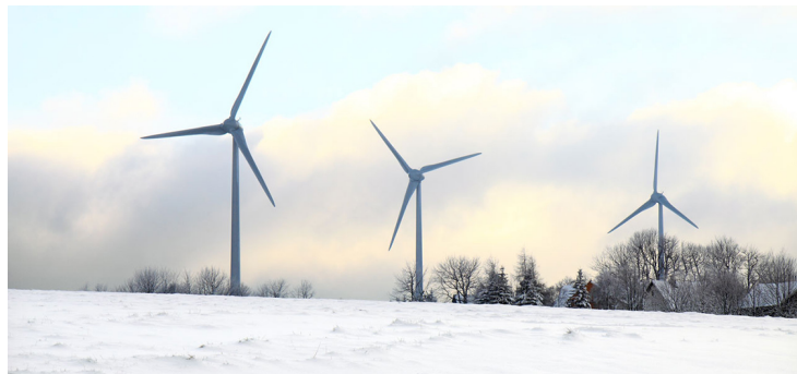
Figure 8.1.1: These wind turbines in the Thames Estuary in the UK are an example of induction at work. Wind pushes the blades of the turbine, spinning a shaft attached to magnets. The magnets spin around a conductive coil, inducing an electric current in the coil, and eventually feeding the electrical grid. (credit: modification of work by Petr Kratochvil)
