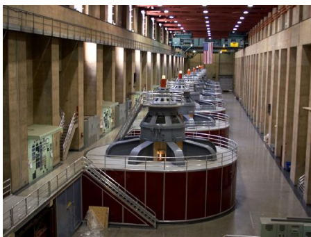
Hydroelectric generators at the Hoover dam. (credit: Jon Sullivan)
