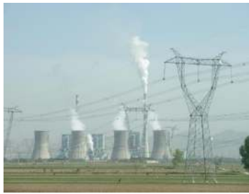
Figure 8.4.4.3: Tremendous amounts of electric power are generated by coal-fired power plants such as this one in China, but an even larger amount of power goes into heat transfer to the surroundings. The large cooling towers here are needed to transfer heat as rapidly as it is produced. The transfer of heat is not unique to coal plants but is an unavoidable consequence of generating electric power from any fuel—nuclear, coal, oil, natural gas, or the like. (credit: Kleinolive, Wikimedia Commons)
