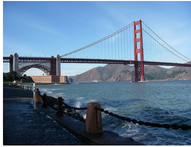
Figure 10.6.4: Unless an infinite tension is exerted, any flexible connector—such as the chain at the bottom of the picture—will sag under its own weight, giving a characteristic curve when the weight is evenly distributed along the length, known as a catenary curve. Suspension bridges—such as the Golden Gate Bridge shown in this image—are essentially very heavy flexible connectors. The weight of the bridge is evenly distributed along the length of flexible connectors, usually cables, which take on the characteristic shape. (credit: Leaflet, Wikimedia Commons)
