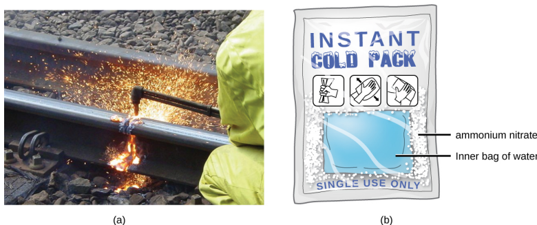
Figure 8.2.8: (a) An oxyacetylene torch produces heat by the combustion of acetylene in oxygen. The energy released by this exothermic reaction heats and then melts the metal being cut. The sparks are tiny bits of the molten metal flying away. (b) A cold pack uses an endothermic process to create the sensation of cold. (credit a: modification of work by “Skatebiker”/Wikimedia commons).
