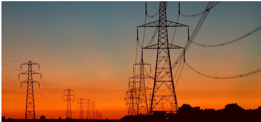
Figure 19.1.1: The current we draw into our houses is an alternating current (ac). Power lines transmit ac to our neighborhoods, where local power stations and transformers distribute it to our homes. In this chapter, we discuss how a transformer works and how it allows us to transmit power at very high voltages and minimal heating losses across the lines.
