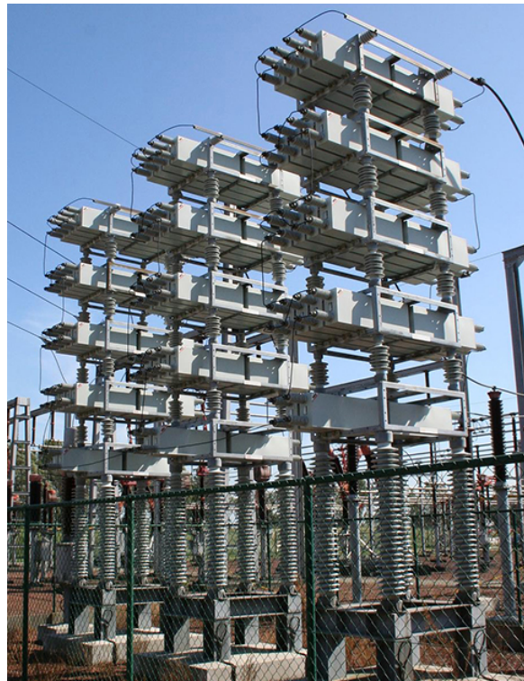
Figure 19.4.4: Power capacitors are used to balance the impedance of the effective inductance in transmission lines.
