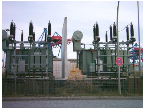
Figure 5.7.4: Power is distributed over large distances at high voltage to reduce power loss in the transmission lines. The voltages generated at the power plant are stepped up by passive devices called transformers (see Transformers) to 330,000 volts (or more in some places worldwide). At the point of use, the transformers reduce the voltage
