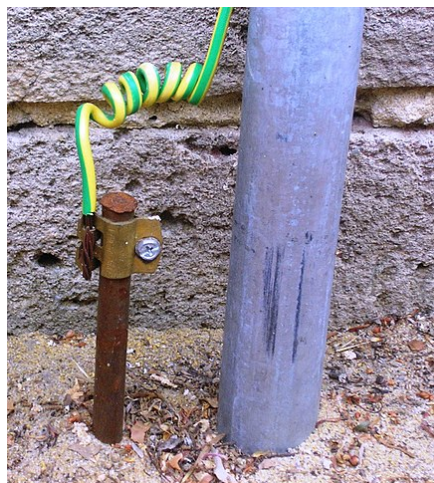
Figure 4.5.1: Example of grounding. The electrical circuits from a building are connected by a conductor (green and yellow wire) into a metal stake into the ground. [3]
