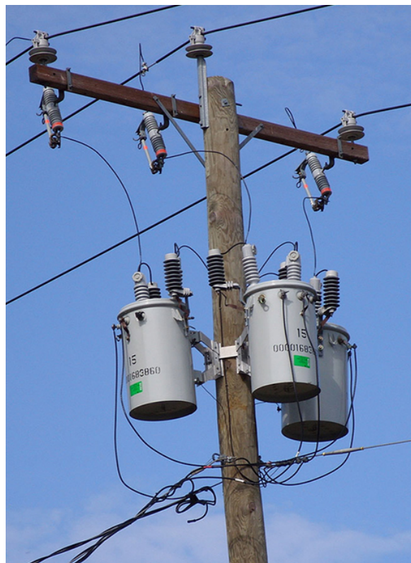
Figure 9.9.2: Transformers are used to step down the high voltages in transmission lines to the 110 to 220 V used in homes. (credit: modification of work by “Fortyseven”/Flickr)
