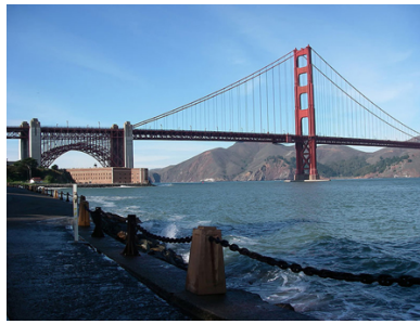
Figure 4.6.4: Unless an infinite tension is exerted, any flexible connector—such as the chain at the bottom of the picture—will sag under its own weight, giving a characteristic curve when the weight is evenly distributed along the length, known as a catenary curve. Suspension bridges—such as the Golden Gate Bridge shown in this image—are essentially very heavy flexible connectors. The weight of the bridge is evenly distributed along the length of flexible connectors, usually cables, which take on the characteristic shape. (credit: Leaflet, Wikimedia Commons)
