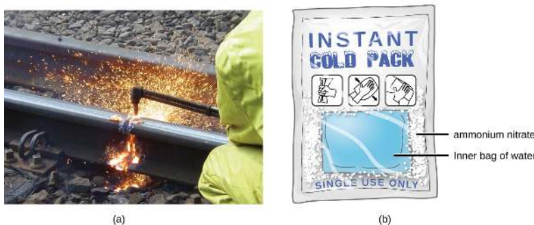
Figure 5.2.8: (a) An oxyacetylene torch produces heat by the combustion of acetylene in oxygen. The energy released by this exothermic reaction heats and then melts the metal being cut. The sparks are tiny bits of the molten metal flying away. (b) A cold pack uses an endothermic process to create the sensation of cold. (credit a: modification of work by “Skatebiker”/Wikimedia commons).
