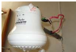
Figure 7.E. 8: On-demand electric hot water heater. Heat is supplied to water only when needed. (credit: aviddavid, Flickr)
