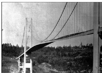
Figure 10.7.4: In 1940, the Tacoma Narrows Bridge in Washington state collapsed. Heavy cross winds drove the bridge into oscillations at its resonant frequency. Damping decreased when support cables broke loose and started to slip over the towers, allowing increasingly greater amplitudes until the structure failed (credit: PRI's Studio 360 , via Flickr)
